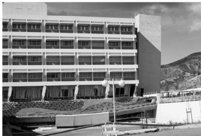
**FIGURE 13.5** Permanent offset of weak first story due to discontinued wall, Olive View Hospital, 1971 San Fernando earthquake. (Photograph by K. Steinbrugge, used with permission from the National Information Service for Earthquake Engineering, University of California, Berkeley.)
